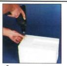
**4.** □ Drill a 1/8" hole through column and attach trim panel to the column with a No. 8 x 3/4" Lg. Phillips flat head stainless sheet metal screw furnished. Follow the same procedure on all four sections.
